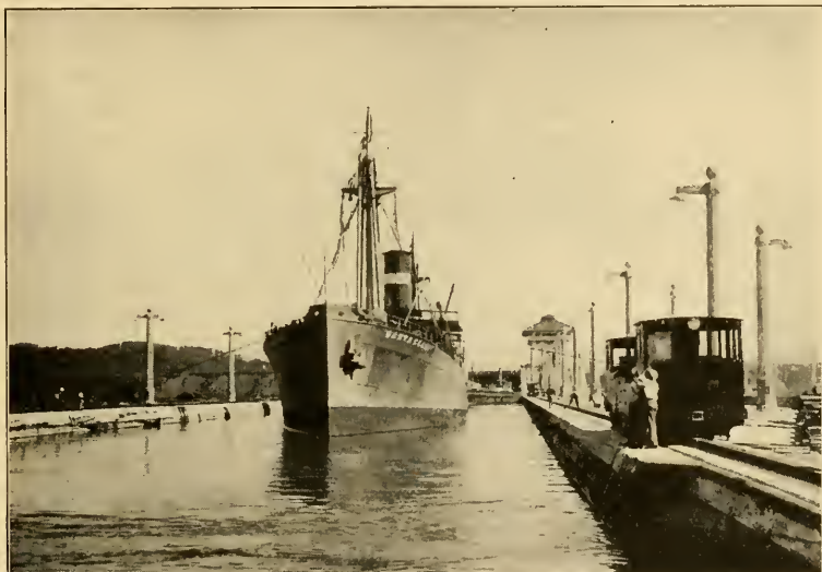
PANAMA CANAL: at the Ninafiores Locks, looking north, showing S. S. Santa Clara in lower west chamber, ready for water to be lowered to sea level.
